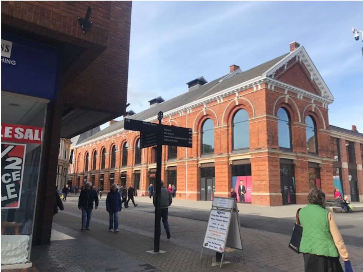
The refurbished Corn Exchange building and new hard landscaping works to the North side of the public realm. The overhang of the 1 st floor of the Cornhill Pavement buildings can be seen to the left.
